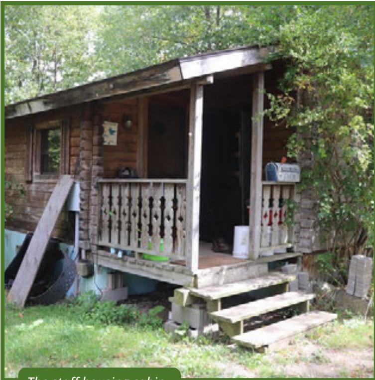
The staff housing cabin.
