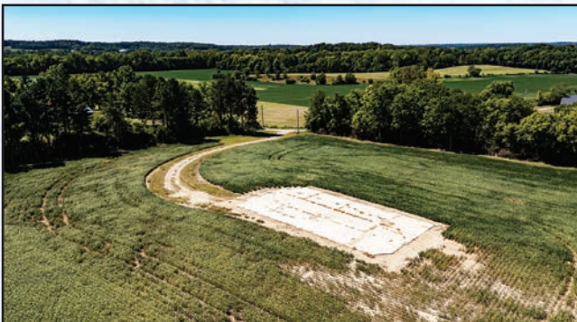
LARGE CONCRETE PAD
