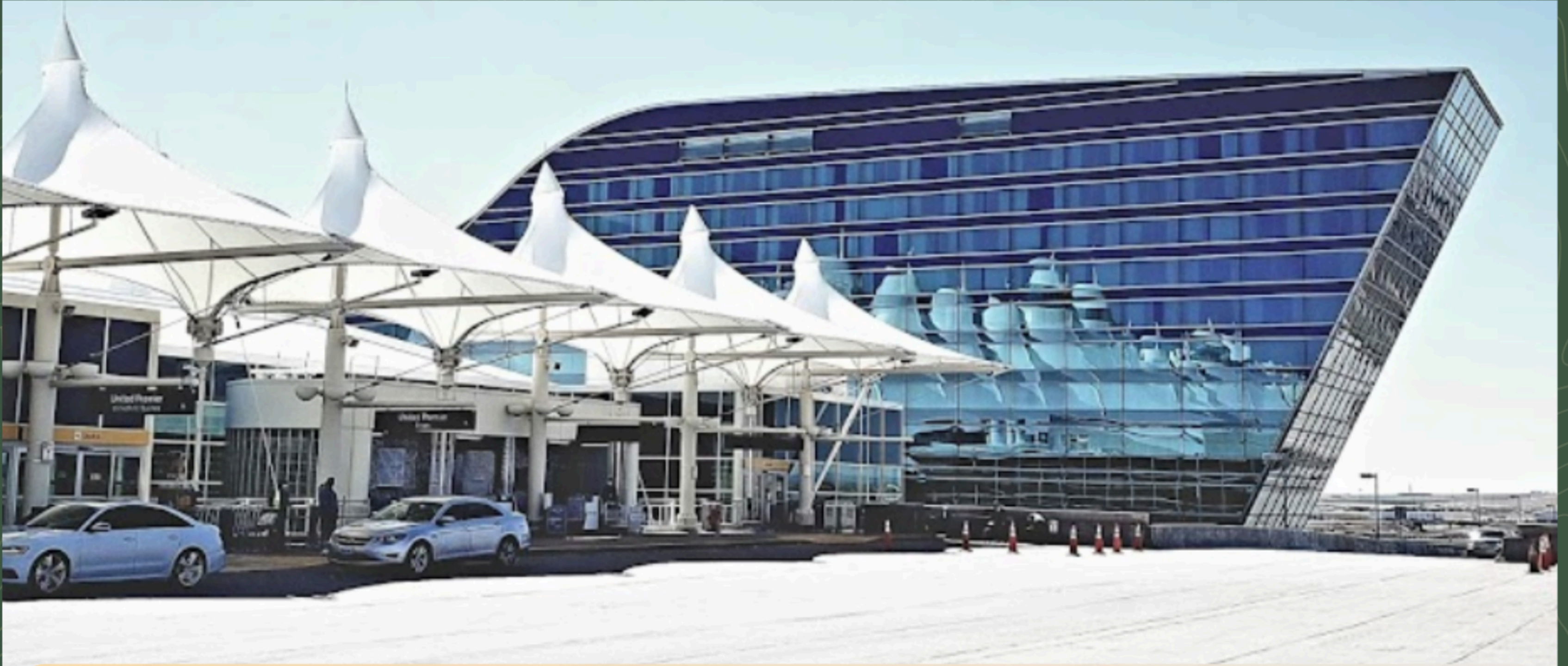
Denver International Airport
